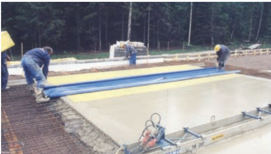
Fig. 2 The top cover is unrolled over the filter pads.
