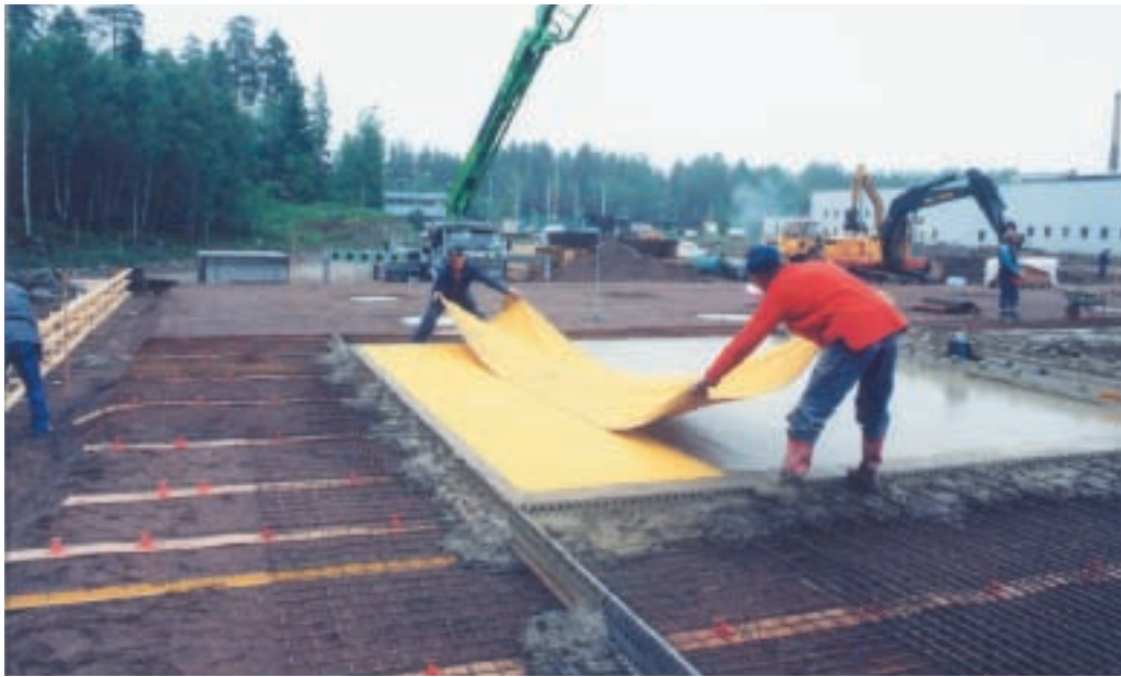
Fig. 1 The filter pads are placed so that there will be a sealing edge around the entire filter pad surface
