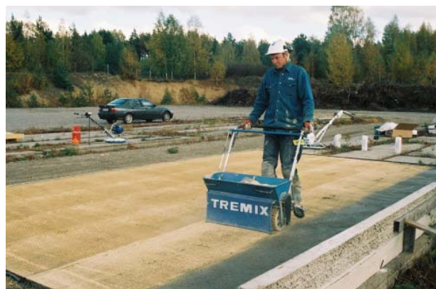
The distribution is easily and evenly carried out with the Tremix spreader wagon TV 830.
